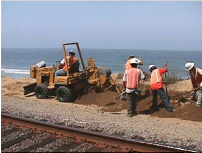
The construction crew digs trenches for sensor cables.
