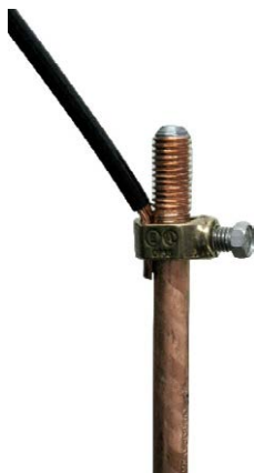
FIGURE 5-14. The #4 cable connected to the ground rod
