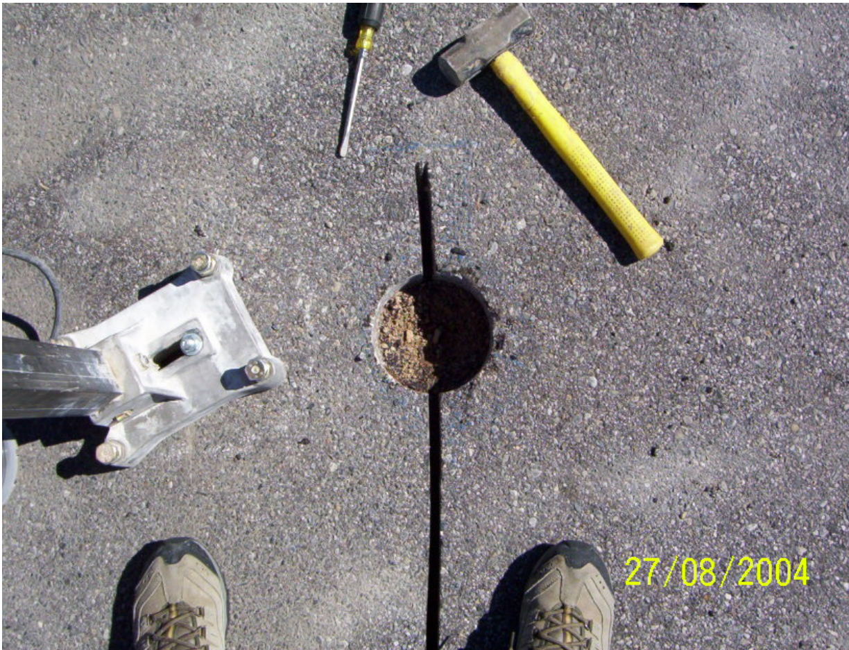
FIGURE 3-1. Core cut for the road sensor.
