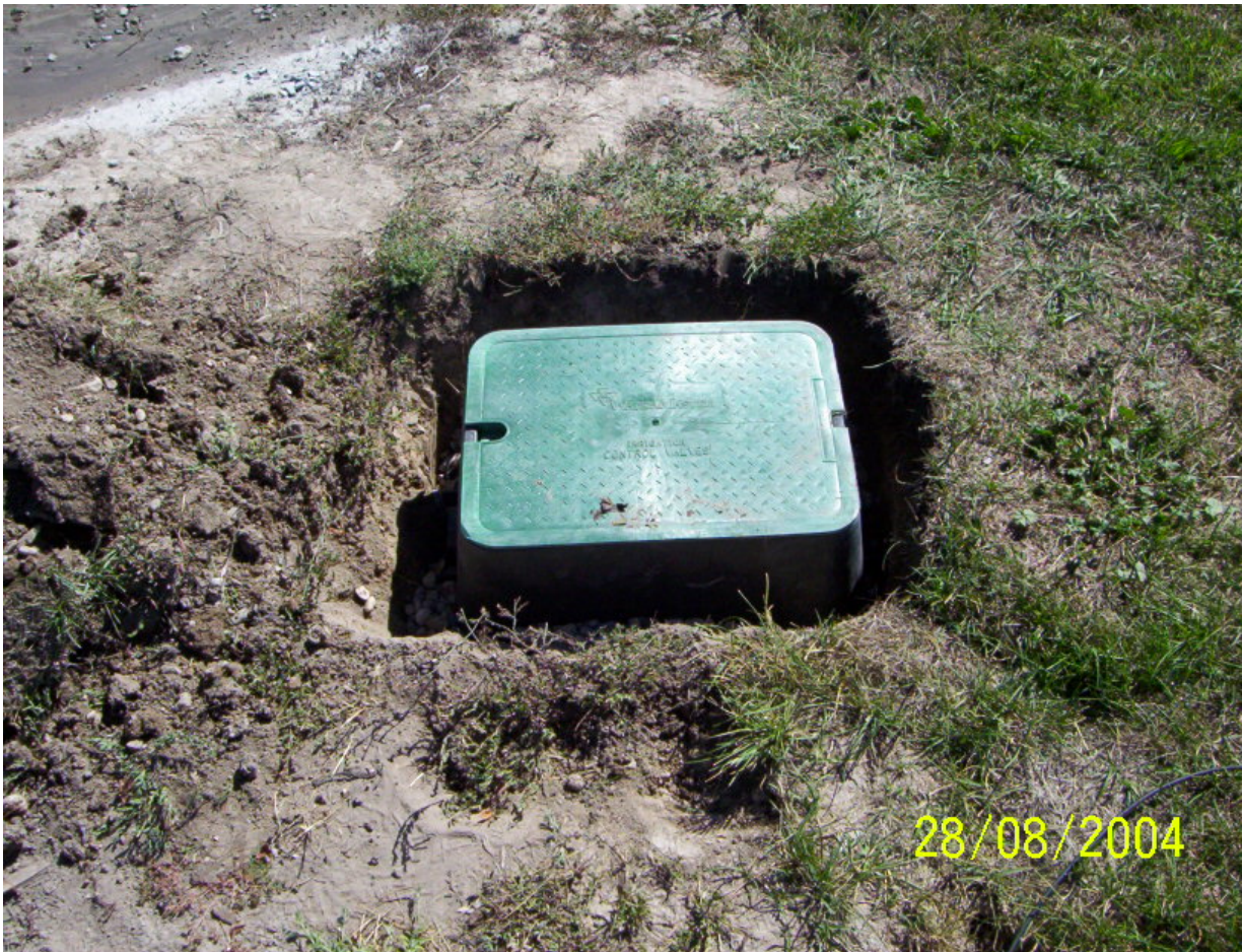
FIGURE 3-13. A junction box is used when cable splices are needed to extend the cable length.
