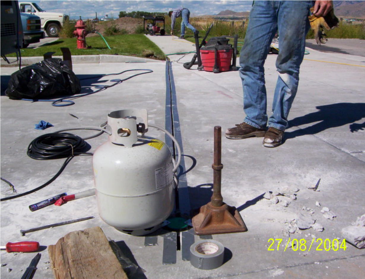
FIGURE 3-3. Saw cut is masked with duct tape to control the epoxies.
