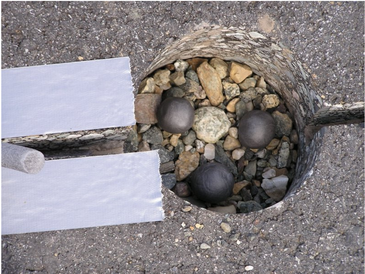
FIGURE 3-4. View of fast steel which is placed under the sensor prior to epoxy application to provide a base for the sensor.
