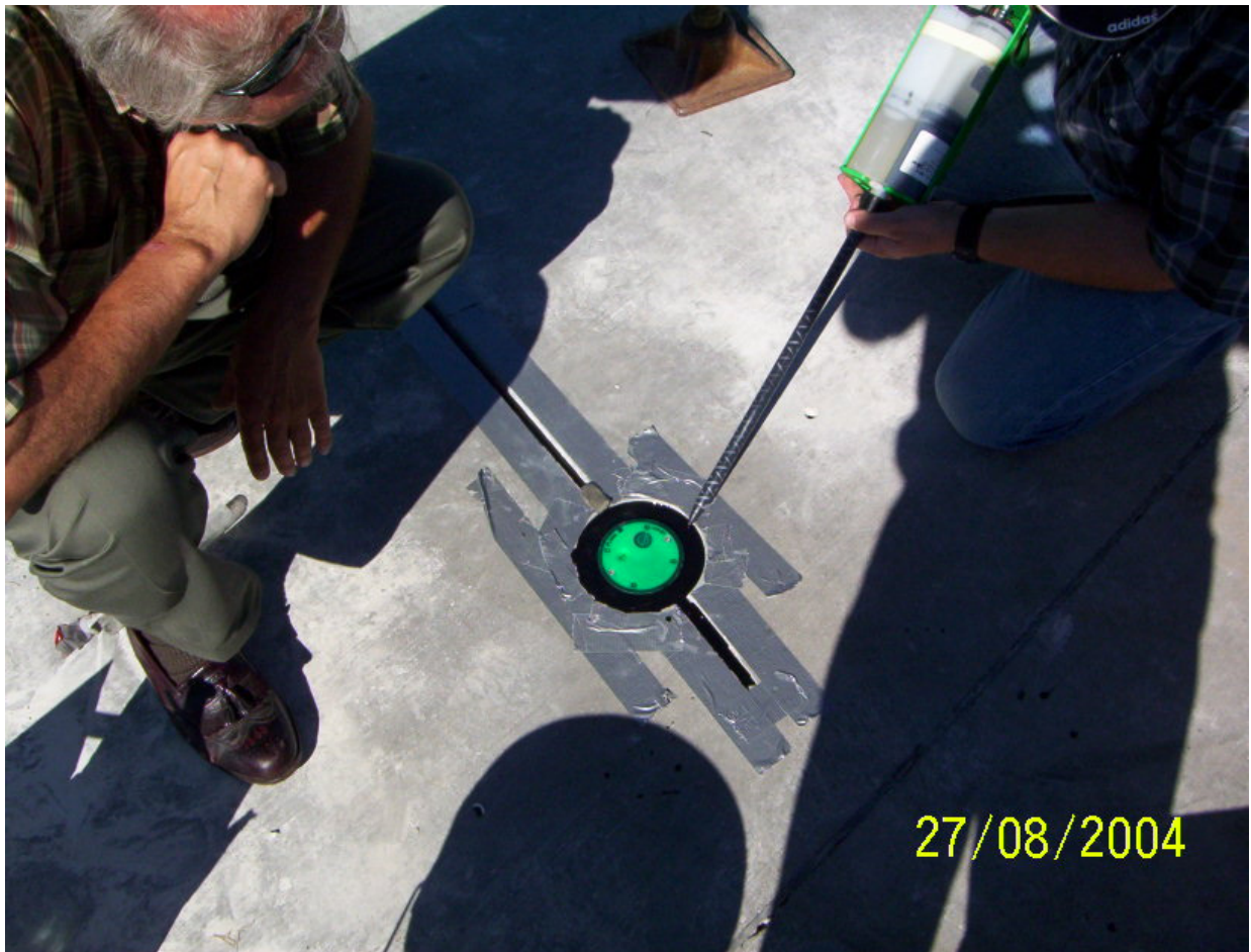
FIGURE 3-8. Second pour to bring the epoxy to grade.
