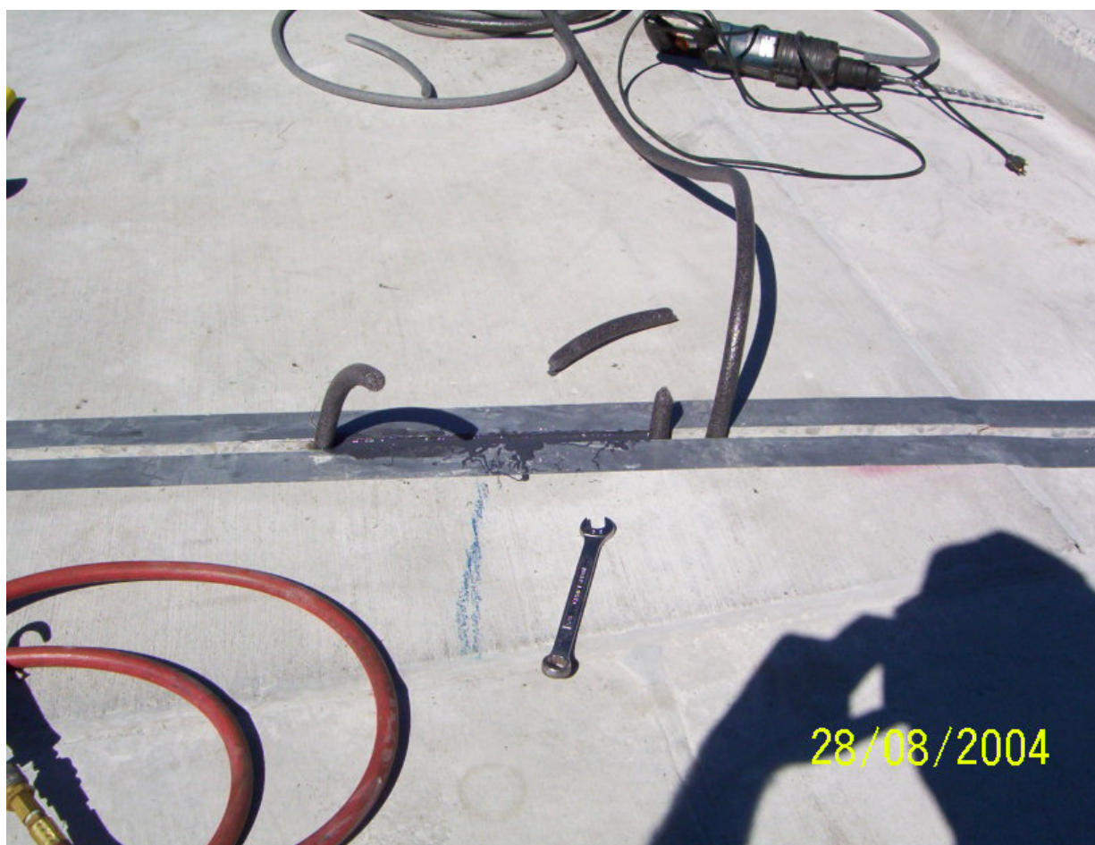
FIGURE 3-9. Backer rod is used as a dam to control the epoxy. Different epoxies can be used for directly around the sensor and along the cable. Since the epoxy used is liquid, the backer rod is used to dam the epoxy until cured.
