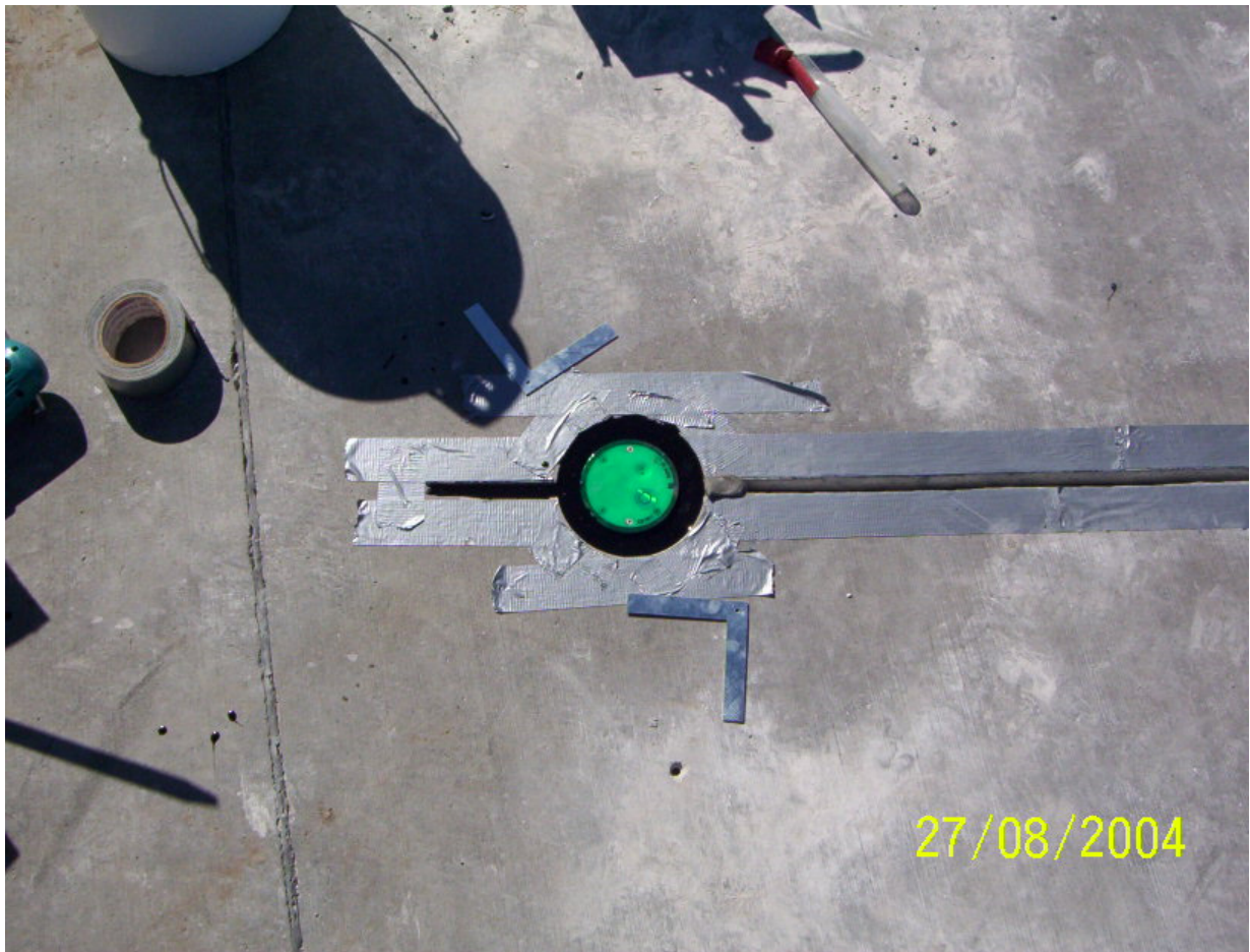
FIGURE 3-12. Finished epoxy application.
