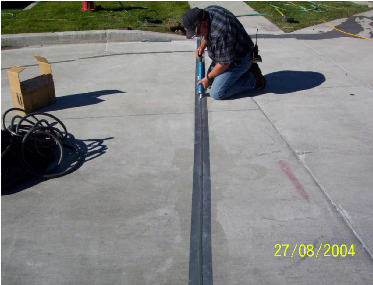
FIGURE 3-11. Application of the sensor cable epoxy. The saw cut is two inches deep. The backer rod is placed in the length of the saw cut below and above the sensor cable before epoxy application.
