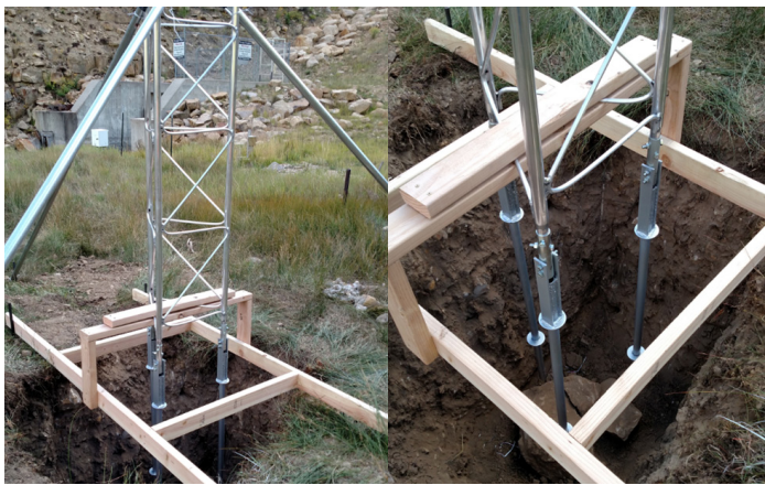
Figure 1: B18 and Tower Installation
