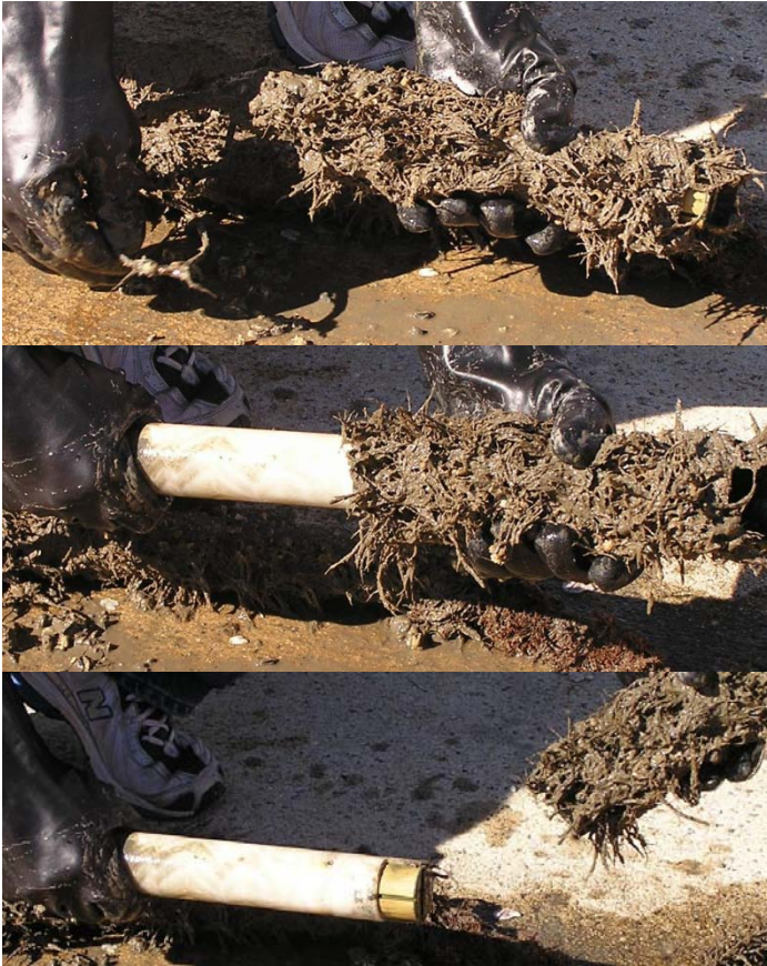
Figure 17. Process of removing a disposable plastic sleeve
