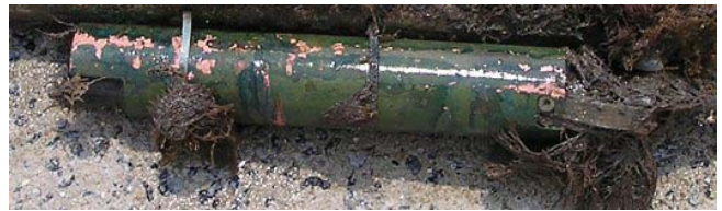
Figure 19. Copper sleeve after 137 days at Skidaway Georgia site
