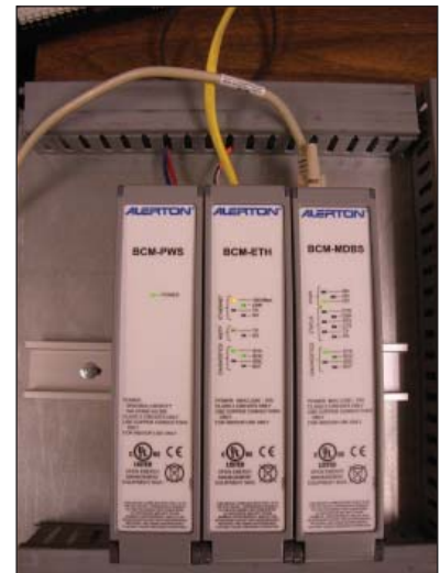
Figure 1. The BCM-PWS, BCM-ETH, and BCM-MDBS modules.
