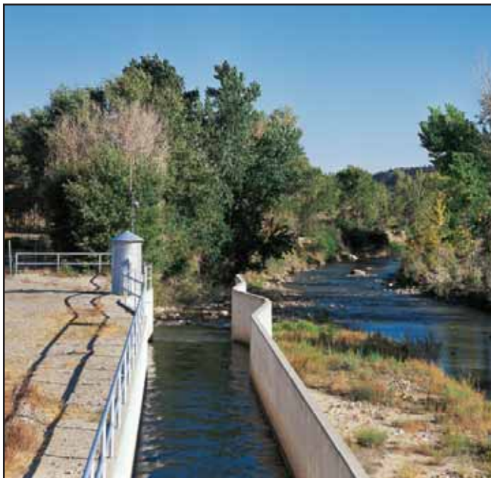
Datalogger measures water level using a shaft encoder, then calculates flow. The data are telemetered, via radio, to the water master for further processing, review, and archive. Stilling well at diversionary dam, Emery County, Utah.
