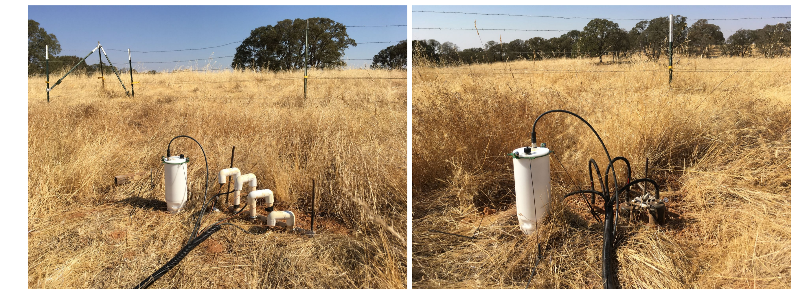
Figure 4: Photos for 2 of 4 eosFD units installed at the Tonzi and Vaira sites in late October, 2017. eosFD units were colocated with gradient measurements for future comparison.
