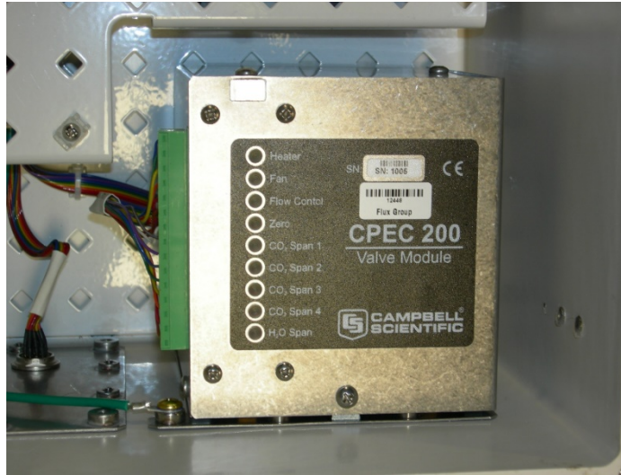
FIGURE 4-8. CPEC200 six-valve module (pn 26578)
