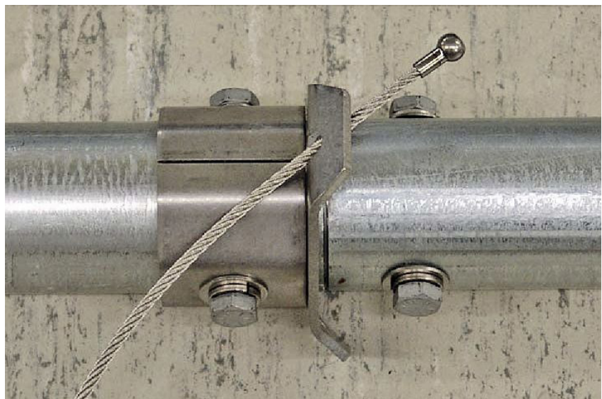
FIGURE 3-16. Mast Section 5 and guy ring/collar assembly
