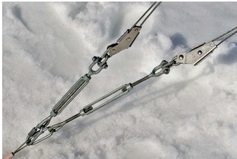
FIGURE 3-26. Top and bottom guy cables fastened to an anchor
