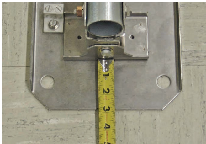
FIGURE 3-20. Tape measure in slot for South anchor
