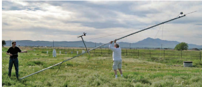
FIGURE 3-29. Raising the mast
