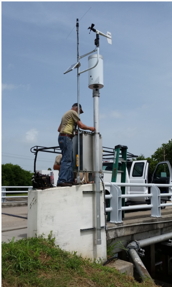
Installing Campbell system for HCFCD
