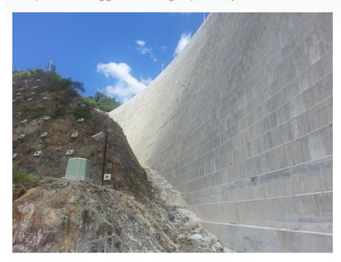
The Portugués Dam is a roller-compacted concrete, thick-arch dam on the Portugués River, 5 km (3 mi) northwest of the city of Ponce, Puerto Rico, USA. Construction on the dam began in April 2008 and finished in February 2014. The dam is 67 m (220 ft) high and 370 m (1,214 ft) long.
