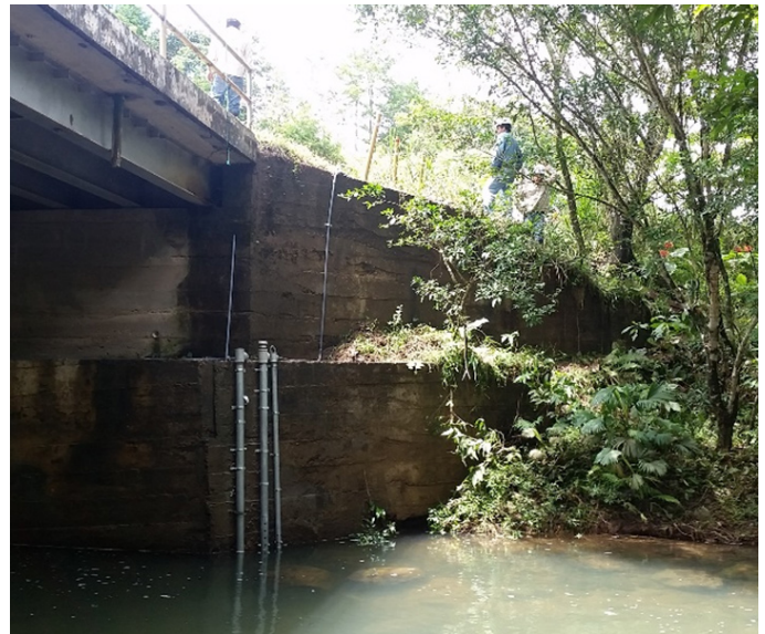
Conduit for the turbidity and conductivity and temperature sensors as well as the sampler hose
