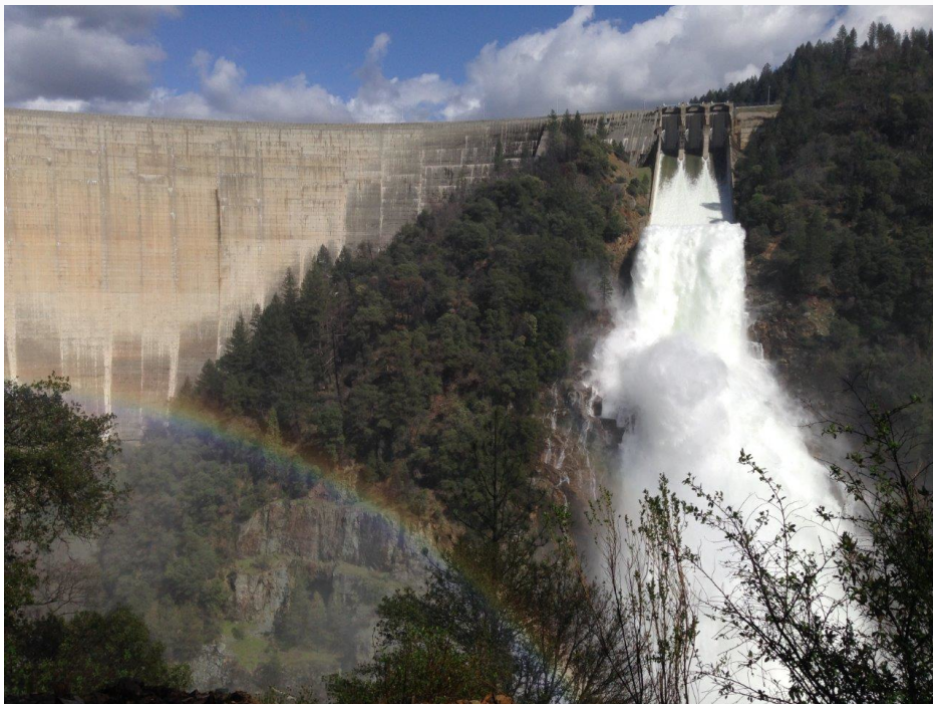
Bullards Bar Dam (Photo courtesy of Charles Johnck)
