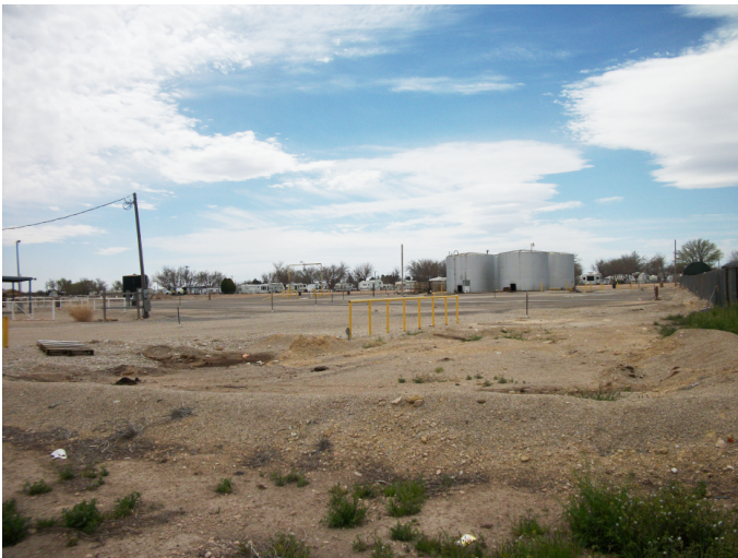
Abandoned brine storage tanks above the cavern
