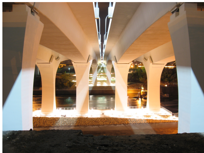
The new St. Anthony Falls Bridge as seen from below (Photo courtesy of Collin Anderson)
