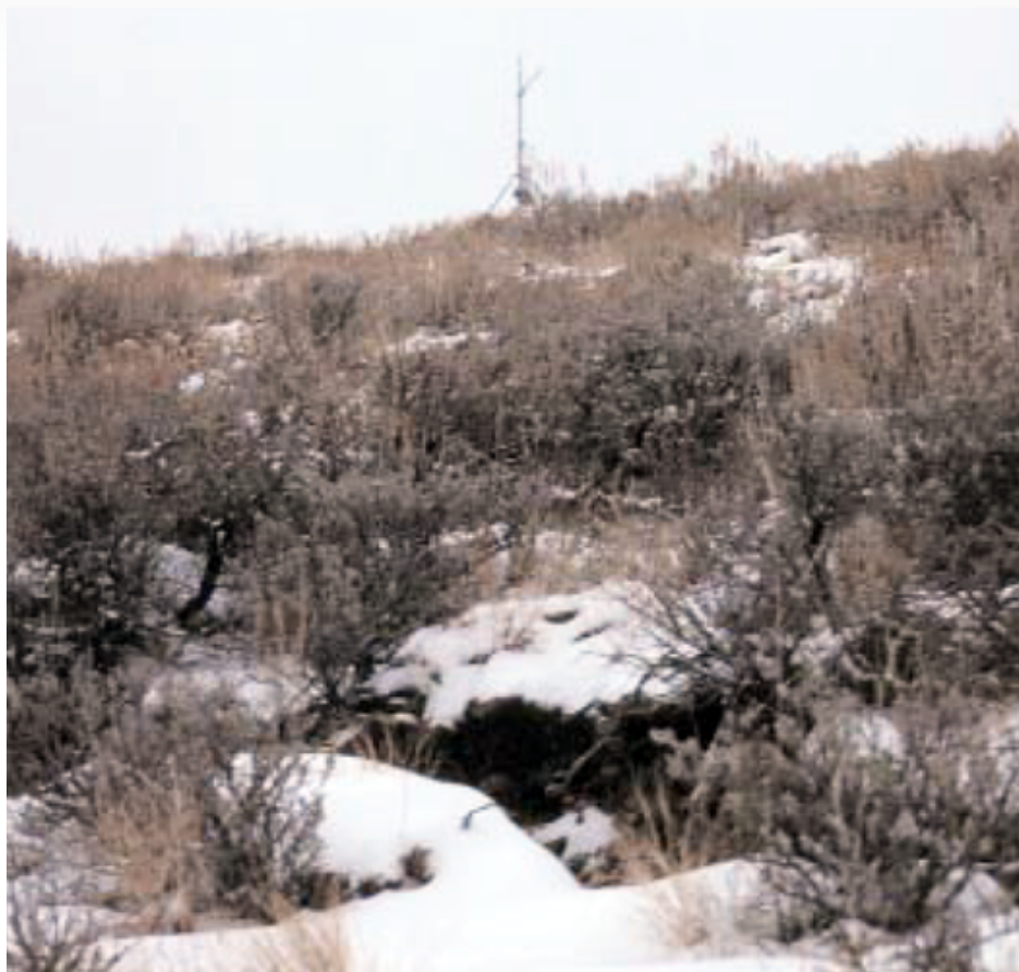
View upslope across fissure system (foreground) to measurement station
