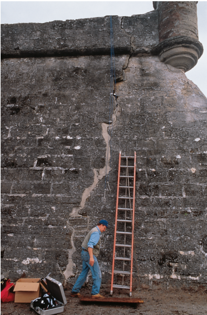
Sensors are installed across a crack in the southwest bastion.
