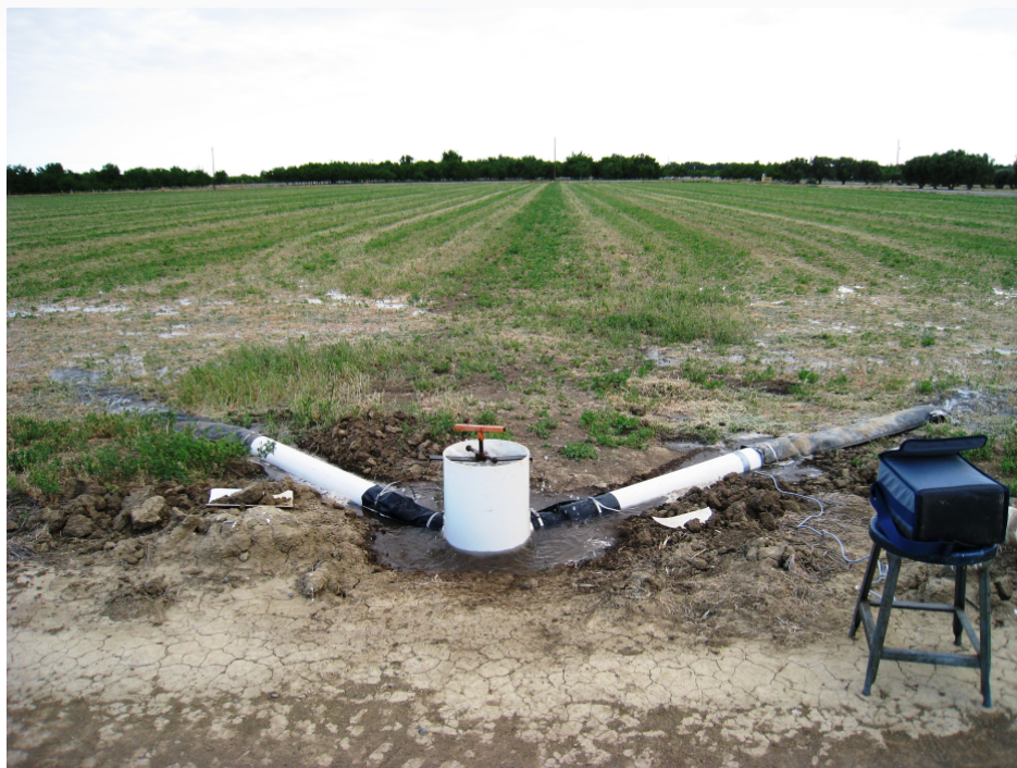
(Photo courtesy of Rajat Saha, MBK Engineers)
