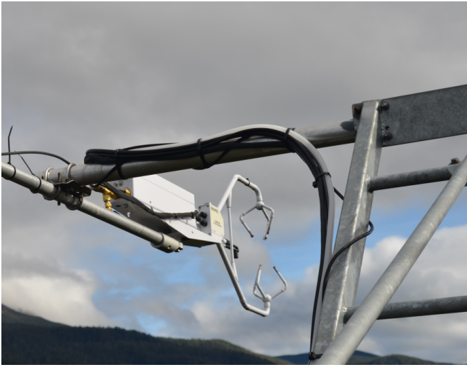
The CPEC200 with vortex intake at the top of the 80-m Warra flux tower
