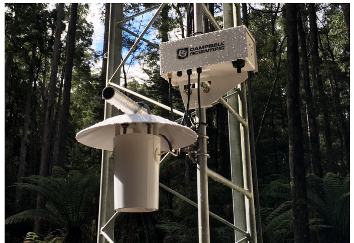
One of the AP200 intakes and the aspirated temperature probes
