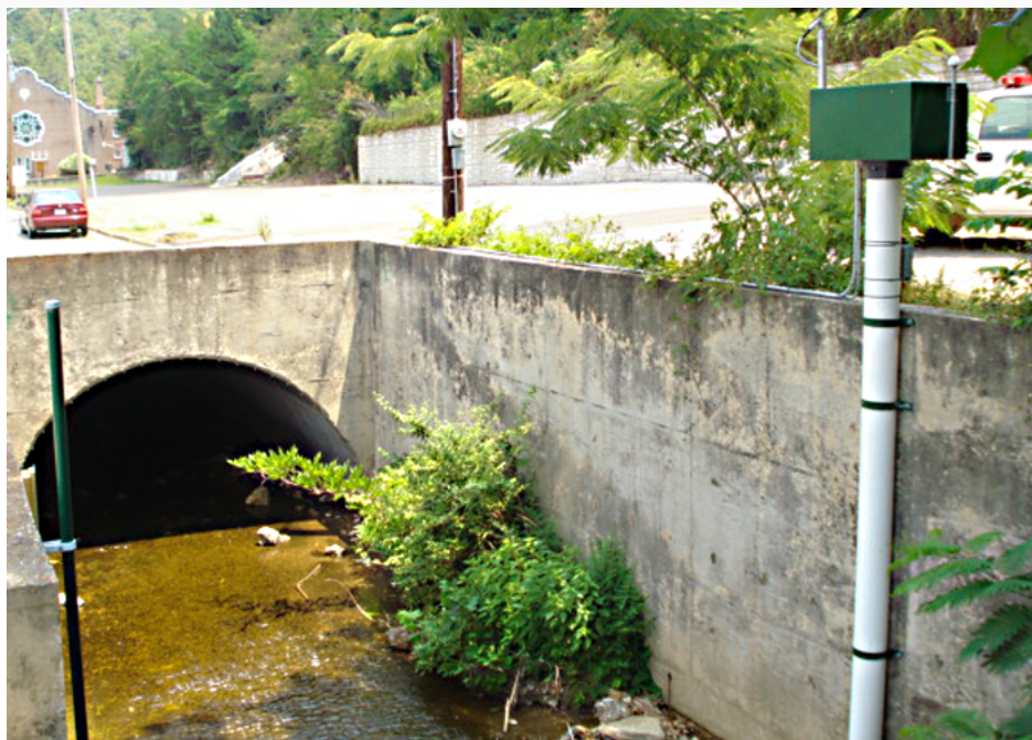
USGS gaging station on Whittington Creek north of Hot Springs
