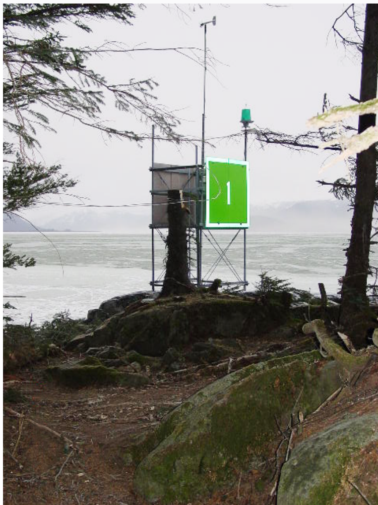
Weather station project installed on the coast of southeastern Alaska
